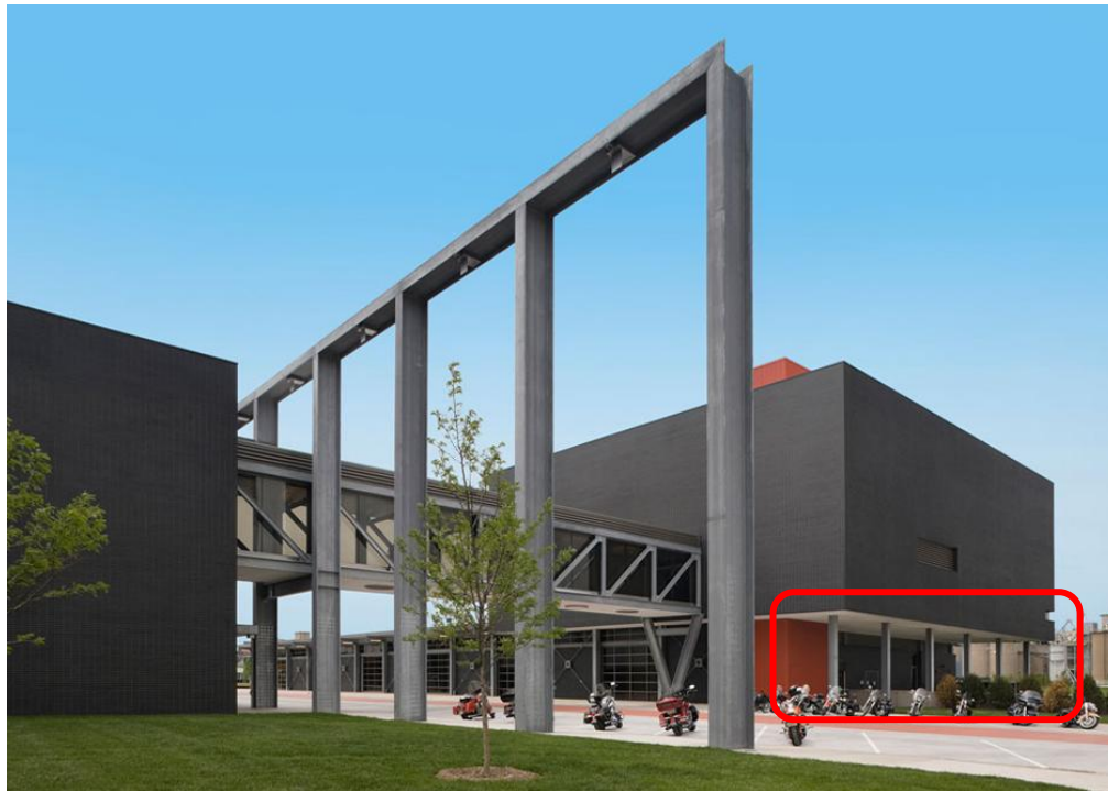
Figure 7 – Columns where thermal bridging is established
