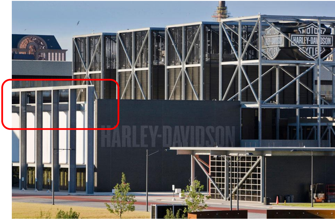
Figure 6 – Beams where thermal bridging is established
